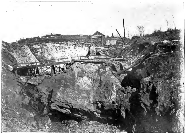
FIG. 86.—View of open-cut at south end of Mine Hill, Franklin Furnace, N. J., exposing the syncline of ore. From a photograph by J. F. Kemp, February 24, 1899.
